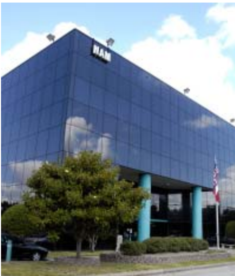
Building Maintenance Endowment Fund reaches $1.0 million.
